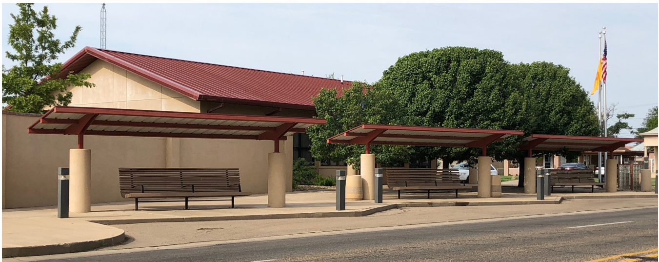
CATS Bus Shelter.
